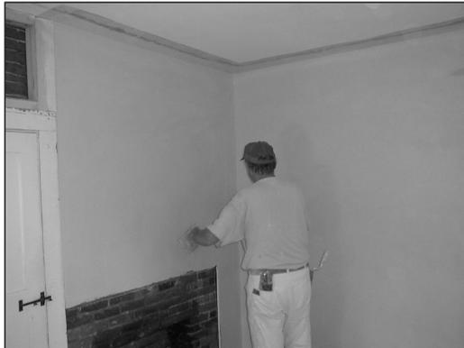
Eugene Zordan applies new plaster to the wall of the 1st floor south bedroom. The original split lath has been incorporated into an exhibit above the door on the left.
