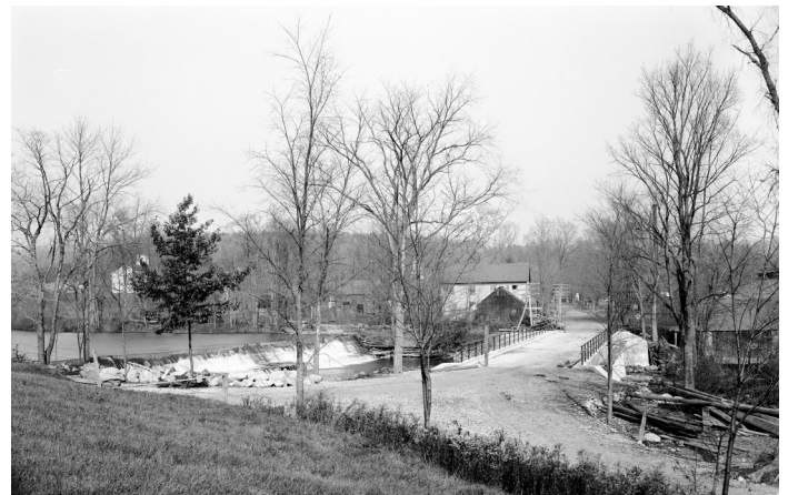
Photo above: one of Mike Day's historic Riverton photos: the bridge over Sandy Brook near the Riverton Grange, circa 1930.
