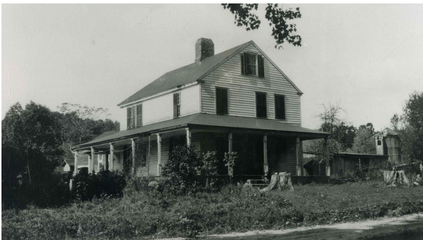
Photo above- a George Merrill farmhouse in Barkhamsted Center.
