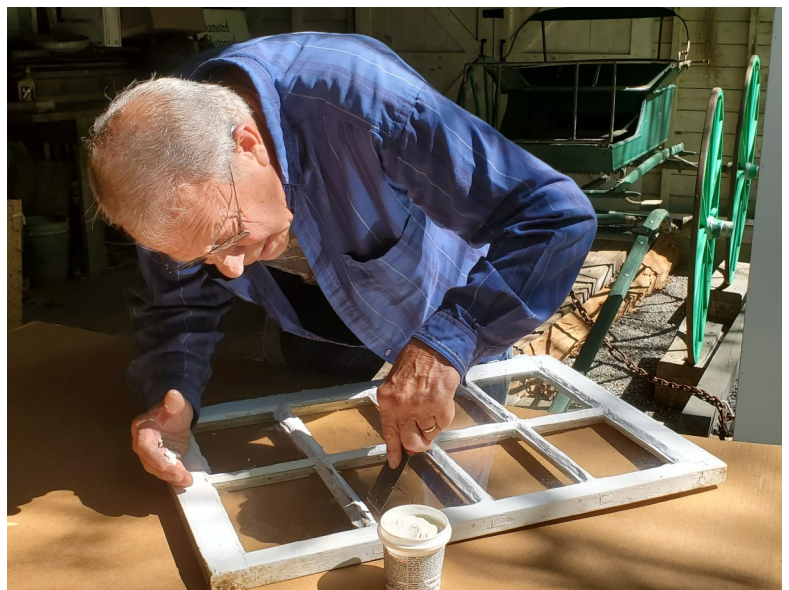
Photo above: BHS volunteer Charlie Watson replaces a broken pane of glass in one of the Squire's Tavern attic windows.
