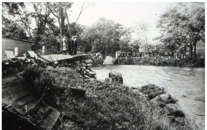
Phot below: Local residents view the damage from the 1938 flood which washed out the old bridge and led to a completely new design for the river crossing here.
